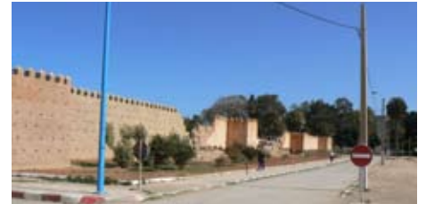
19th century Kasbah currently being restored
